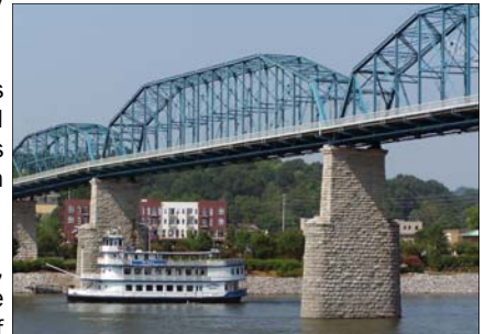
Walnut Street Bridge
